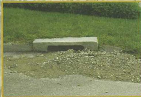
BAD BMP: Debris covers a storm drain interfering with drainage. Dirt is also being allowed in our waterways. This is what we do NOT want to find when we are out on job-site inspections.
